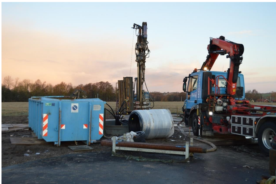
Figure 24. The drilling rig on site, drilling one of the BHEs.
