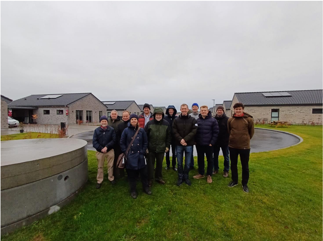
Figure 26. The commissioned Thermo-road with buildings occupied by tenants. The picture was taken during a field site tour with visitors Dr. Matt Mitchell from National Renewable Energy Laboratory (US), Regents Professor Jeffrey Spitler from Oklahoma State University (US), Professors Johan Claesson and Jesper Arfvidsson, and Dr. Akram Habdul Hamid from Lund University (Sweden), CEO Dr. Signhild Gehlin from Svenskt Geoenenergicentrum (Sweden), Dr. Tor Helge Dokka from Skanska (Norway), CEO Søren Skjold Andersen and Bjørn Kassøe Andersen from Geodrilling (DK), senior researcher Viktor Søgaard from GEUS (DK), and finally researcher Kristoffer Bested Nielsen (VIA), Dr. Karl Woldum Torstrup (VIA) and project manager, Head of Research Dr. Søren Erbs Poulsen (VIA).
